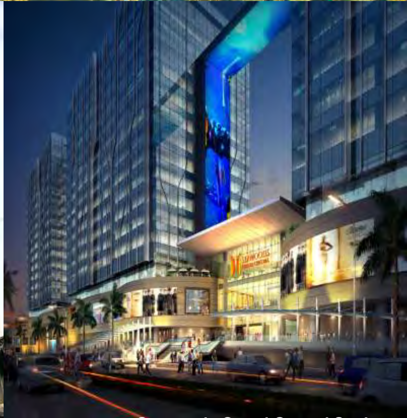
Seawoods Grand Central Station
